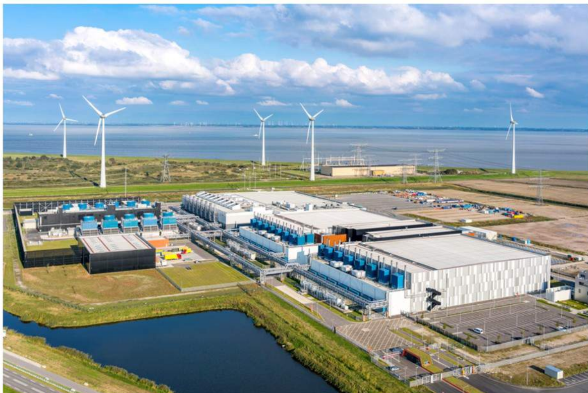
Googles datacenter in Eemshaven
